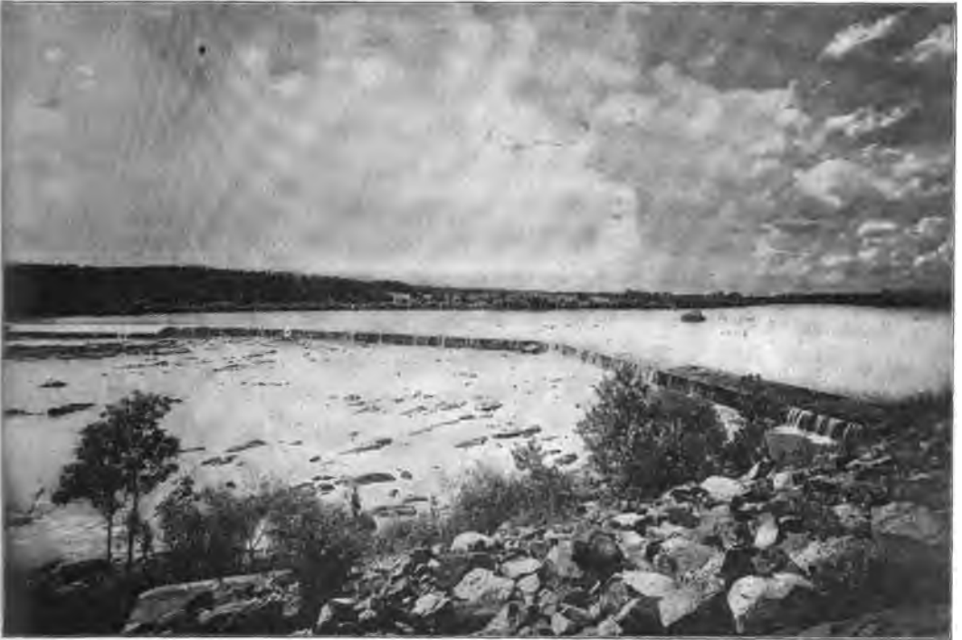
DAM ACROSS BROAD RIVER FOR COLUMBIA CANAL.
